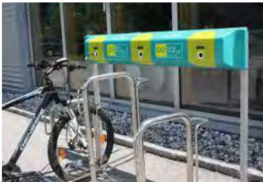
Bsp. Ladestation bike-energy
